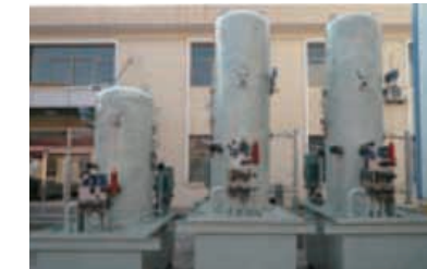
Hydraulic servo-system of governor combined with oil pressure supply unit
