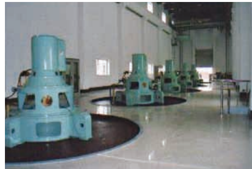
Gate control system for Yantan power station
