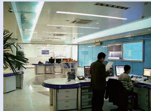
Xining remote control center for the upriver cascaded hydropower station of Yellow River
