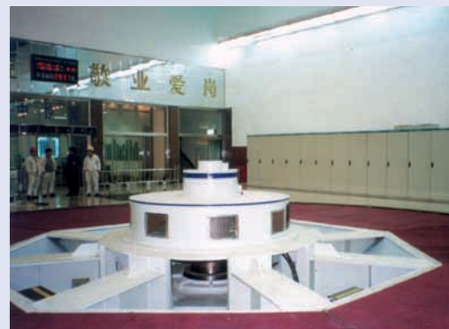
Powerhouse of Dongfeng hydropower station after rehabilitation
