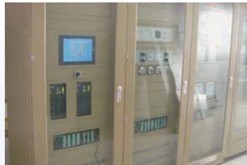
The cubicle of the LCU equipment
