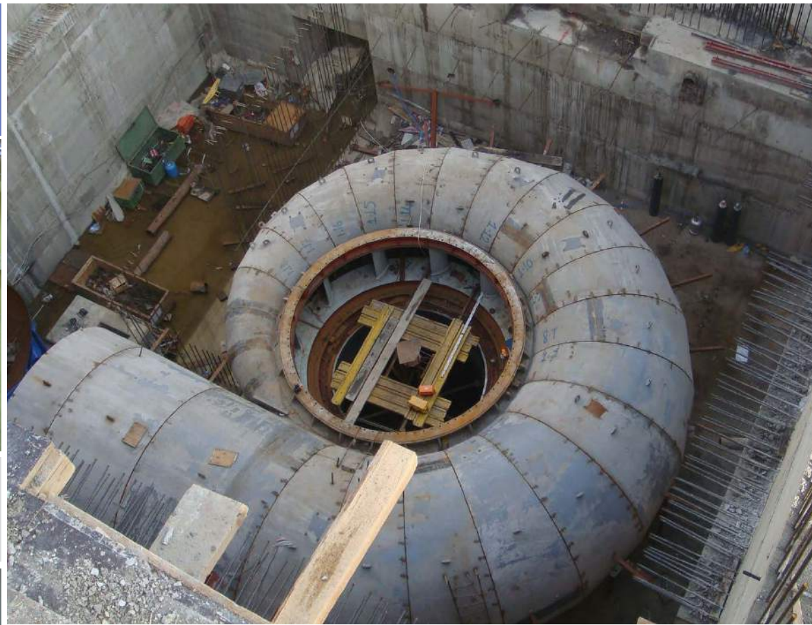
Assembling of scroll case of Bayramhacili Hydropower Station in Turkey
