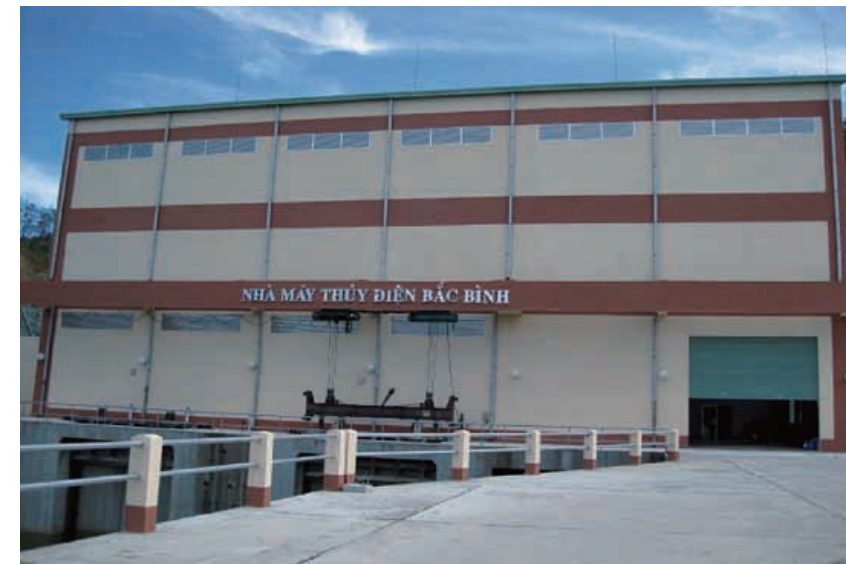
Powerhouse of Bac Binh Hydropower Station in Vietnam
