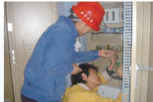
Engineers installing the LCU
