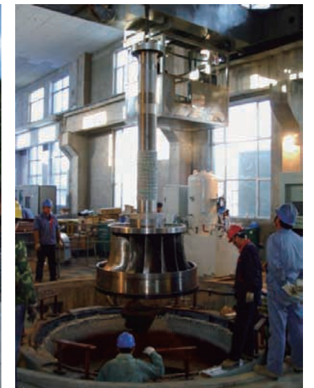
The erection of prototype turbine
