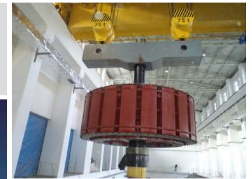
Installing rotor of Gullubag HPP
