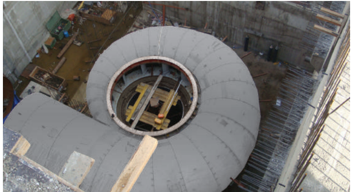
Installing spiral case of Bayramhacılı HPP
